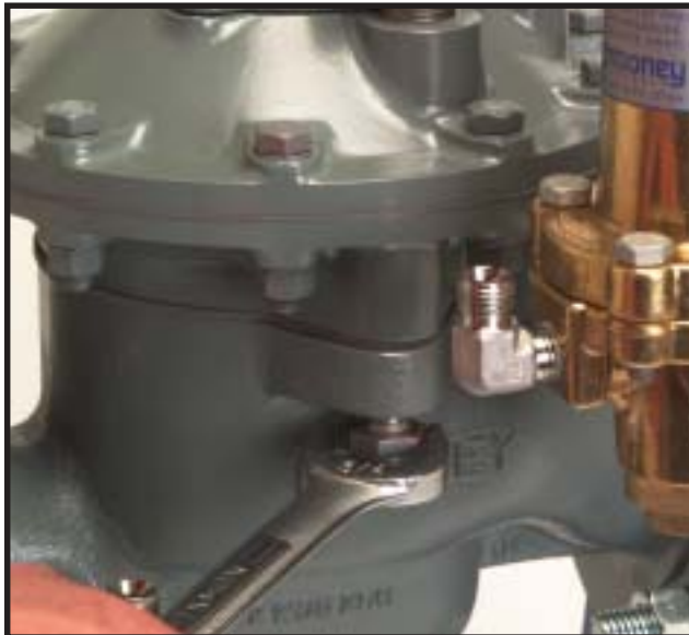
Fig. 27 Tightening the Body Cap Screws
