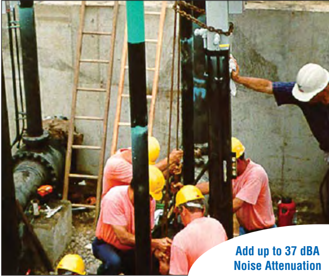
Figure 8 - Installation of Becker Below Ground Ball Valve Regulator.
