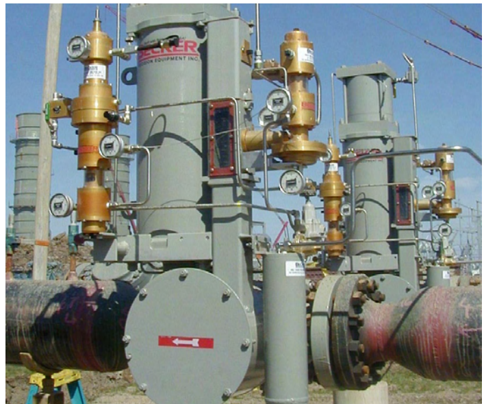
Figure 2.0 – Becker Model QTCV-T1 used as primary regulator in power plant
