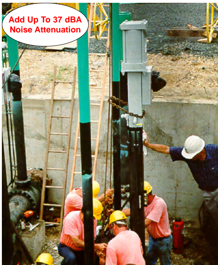
Figure 8.0 Installation of Becker Below Ground Ball Valve Regulator.
