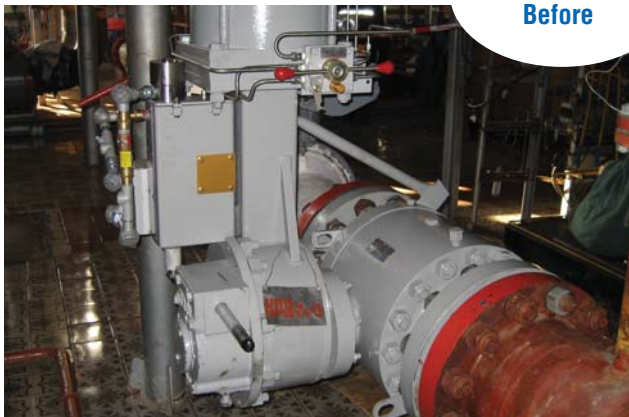
Figure 1 - Typical Becker Control Valve Installation BEFORE Installing ANJ
