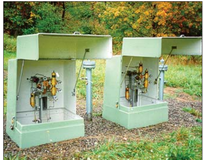
Figure 2 - CAB installed on Becker Below Ground Regulator
